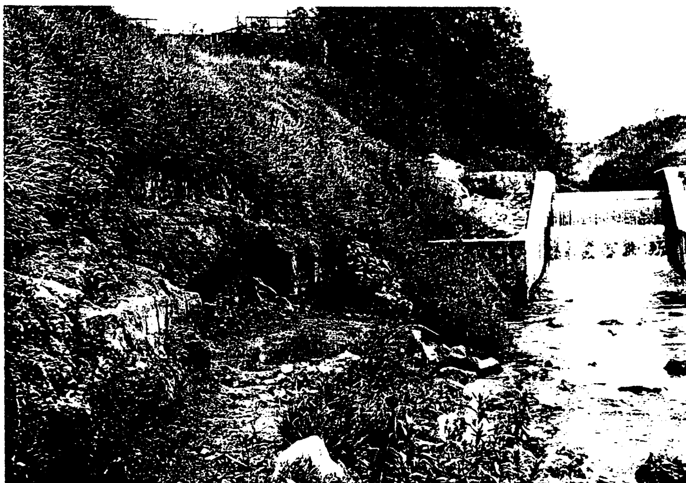
The newly excavated section at Doe Lea immediately downstream from the weir
